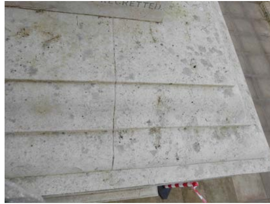
Fig 24: erosion of sky face of moulding
