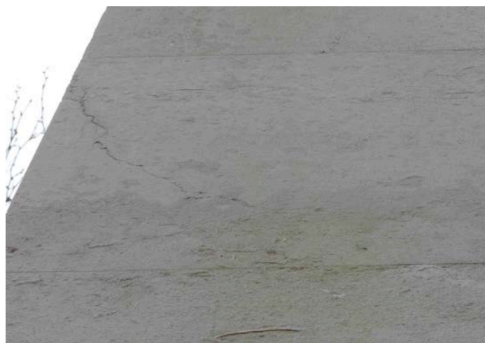
Fig 31: natural fault in obelisk stone
