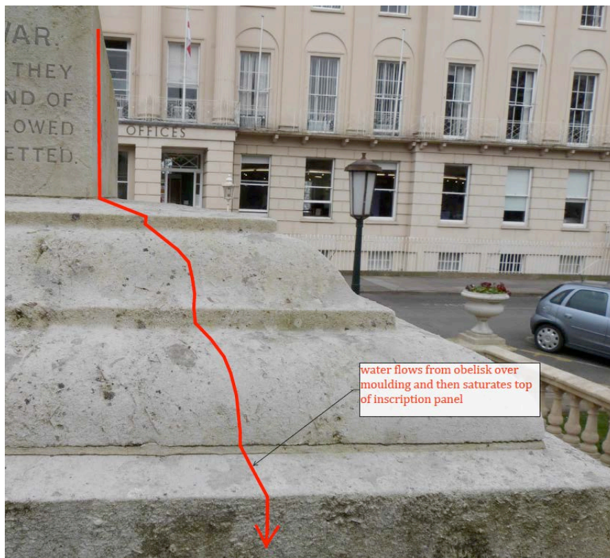
Fig 14: original design leading to saturation of inscription panel
