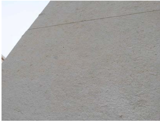
Fig 21: vertical tool marks on obelisk stone
