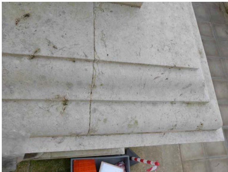
Fig 34: detail of moulding showing cracked joints
