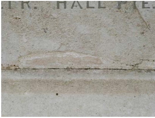
Fig 20: repair at base of inscription panel
