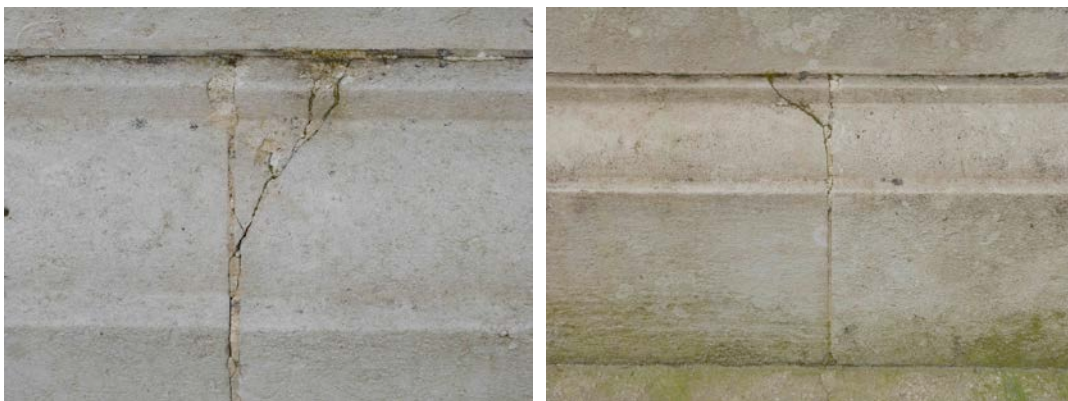
Fig 10 and 11: spalling of base plinth stone due to corrosion of cramps (south and north elevations)
