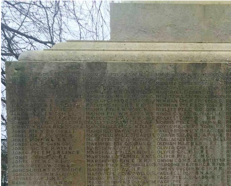
Fig 15: detail of north side inscription panel showing algae growth and how it obscures inscription
