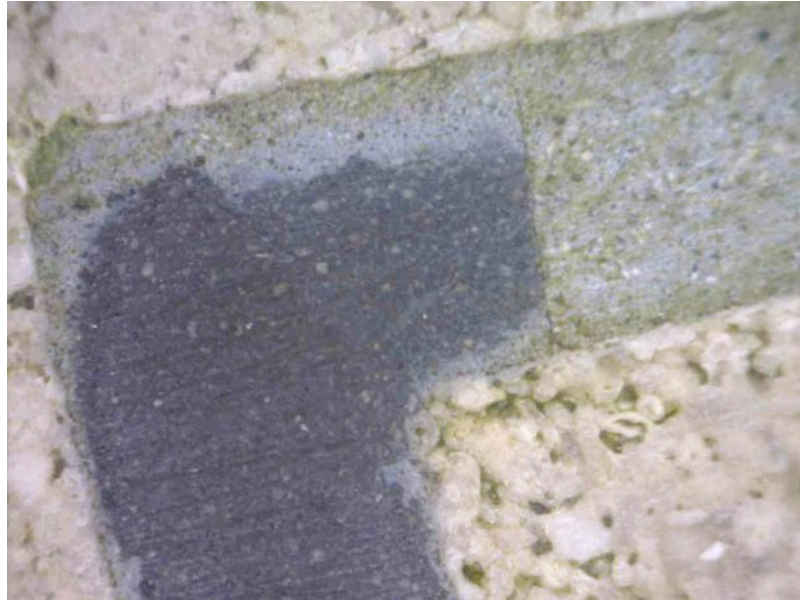
Fig 37: small section of original finish showing dark grey polished appearance
