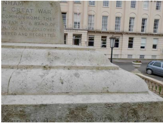
Fig 23: cracked pointing at base of moulding
