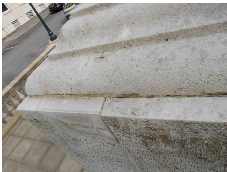
Fig 19: detail of moulding showing cracked pointing
